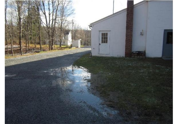
Installing a rain garden in front of the building can capture, treat, and infiltrate roof runoff. Another rain garden can be built to the north of the building to prevent erosion. A preliminary soil assessment suggests that more soil testing would be required before determining the soil's suitability for green infrastructure.
