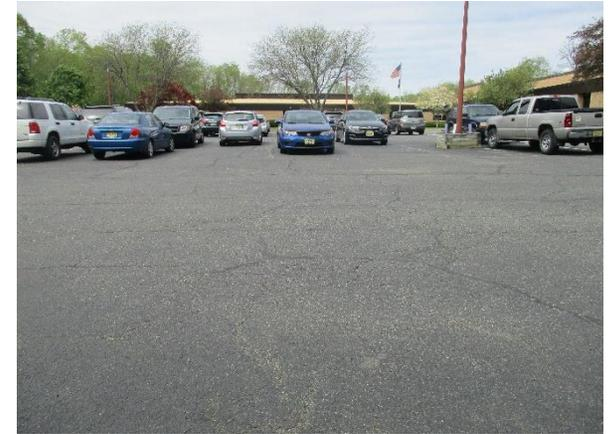
Parking spots to the east of the building can be replaced with porous asphalt to capture and infiltrate stormwater. Installing a rain garden in the back of the building can capture, treat, and infiltrate roof runoff. A preliminary soil assessment suggests that the soils have suitable drainage characteristics for green infrastructure.
