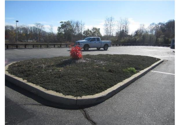
Installing rain gardens in the parking islands will capture, treat, and infiltrate parking lot runoff. A preliminary soil assessment suggests that more soil testing would be required before determining the soil's suitability for green infrastructure.
